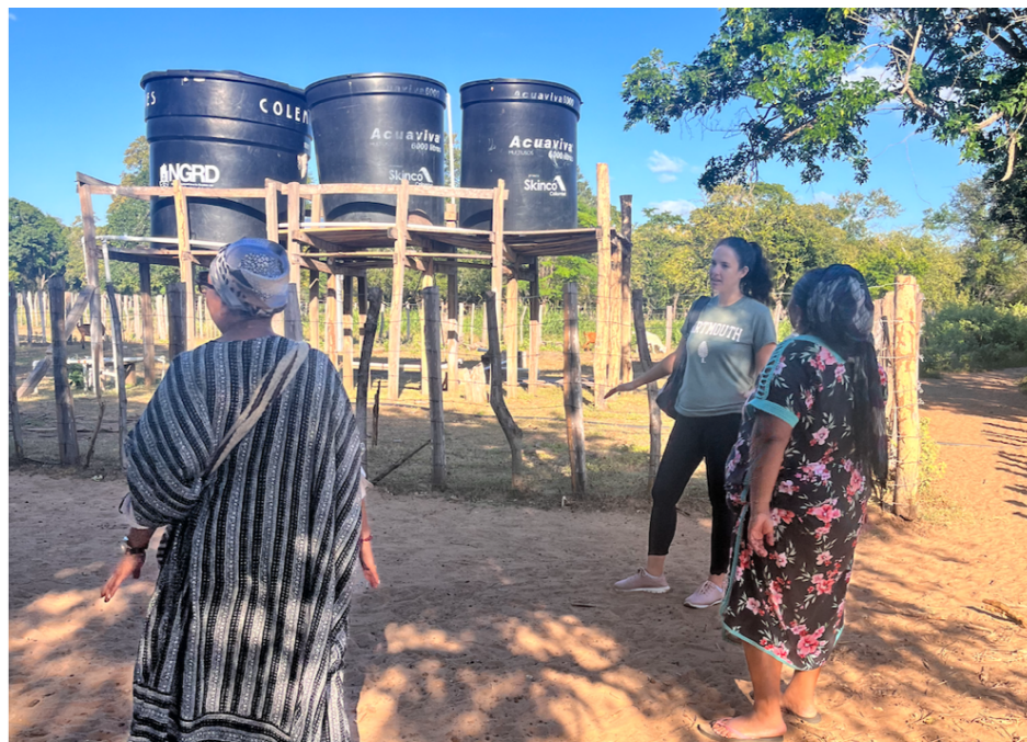
Figure 30 Photo of an irrigation project in Maku (Jan 2023)
