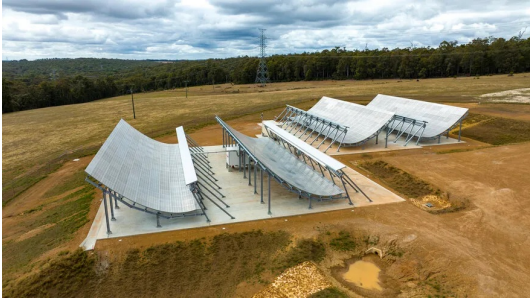
Figure 1: Aerial view of the two S-band active phased array radars at the West Australian Space Radar (WASR) site in Collie Shire, Western Australia.
