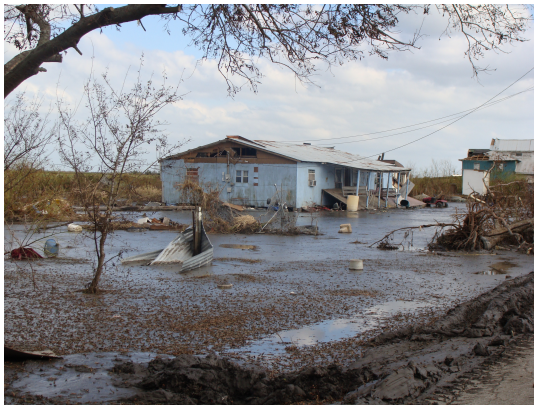
ISLE DE JEAN CHARLES - AUGUST 16, 2007: Southern Louisiana vanishes beneath rising waters.
