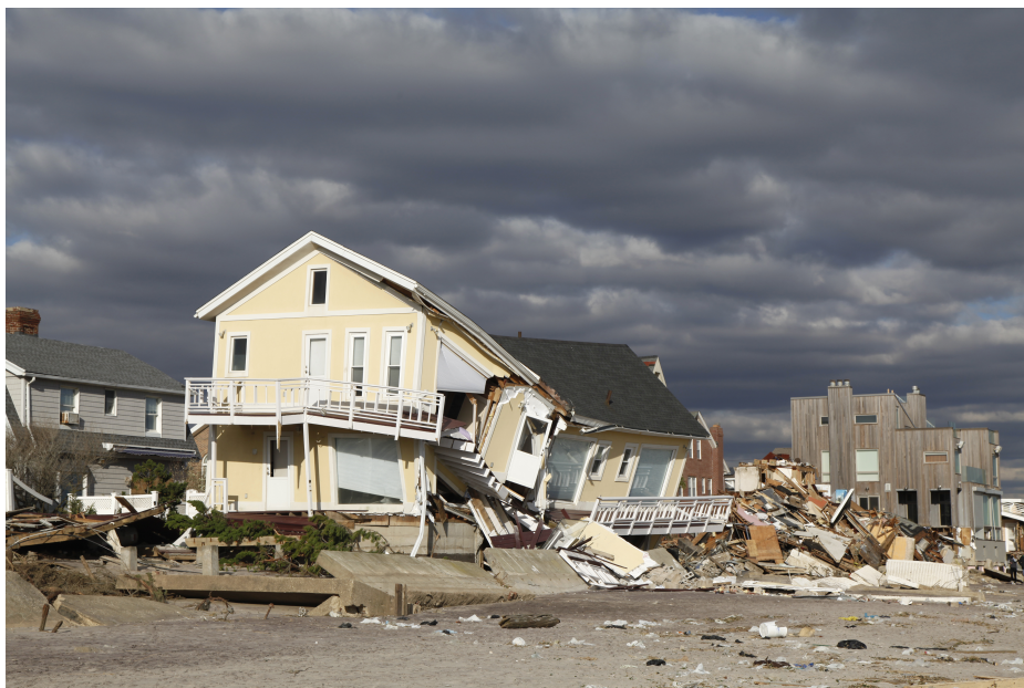
FAR ROCKAWAY, NY - NOVEMBER 4, 2012: Destroyed beach house in the aftermath of Hurricane Sandy
