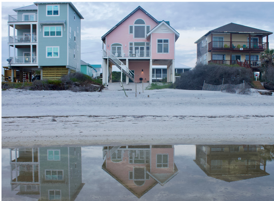
CAPE SAN BLAS, FLA - Elevated beach houses on the Florida Gulf Coast.
