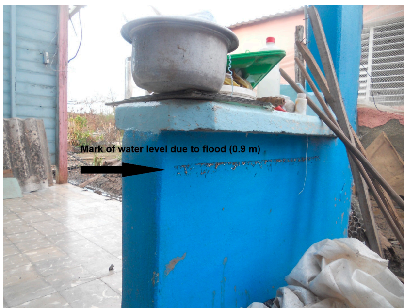
Figure 4. Image of water level (approximately 0.9 m from the ground level) measured at a house in the town of Punta Alegre.
