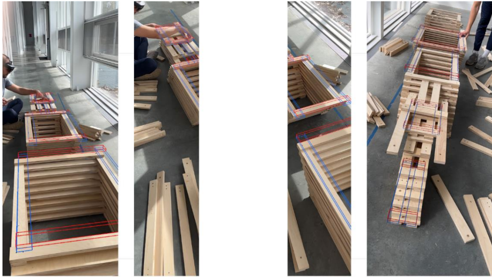
Figure 2. Holographic projection during the assembly
