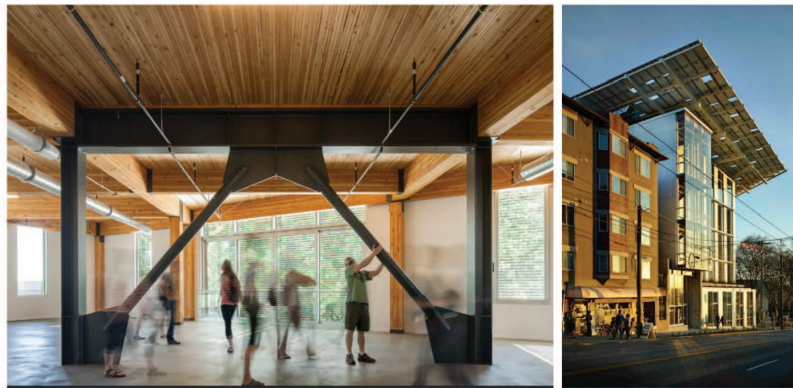
The Bullitt Center in Seattle, Miller Hull Partnership
