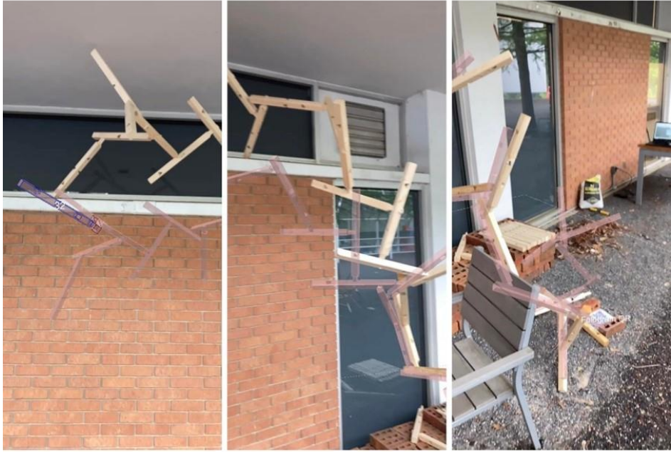
Figure D-13: Holographic projection assisted assembly
