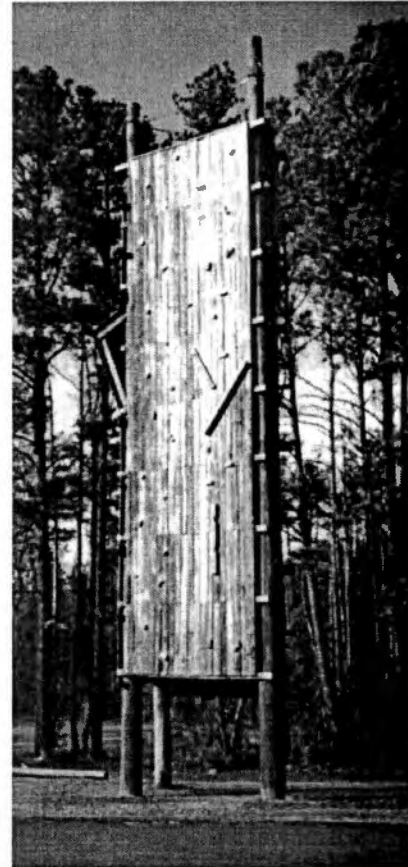
Figure 3.26: Climbing/Rappelling Tower, Project Adventure, Covington, Georgia. A climbing and rappelling wall is often built to complement the sequence of tree-top elements.
