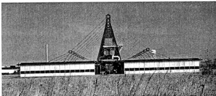
Fig. 2.30. Patcenter Cable Roof Structure. Richard Rogers, architect.
