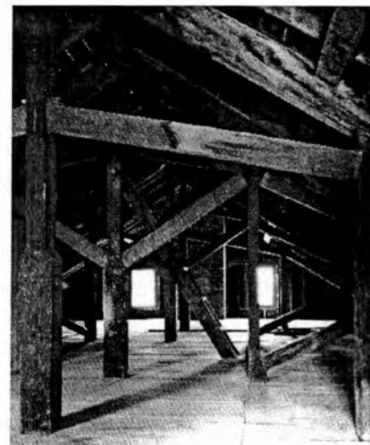
Fig. 2.27: Attic Room, Shaker Village at Pleasant Hill, Ky. Heavy wooden timbers were hewn into load-carrying columns and supports.
