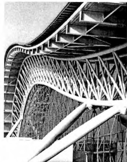
Fig. 2.29: Kansai International Airport, Terminal. Example of steel used as structure, bracing, and cladding. Renzo Piano, architect. Source: Buchanan (144)
