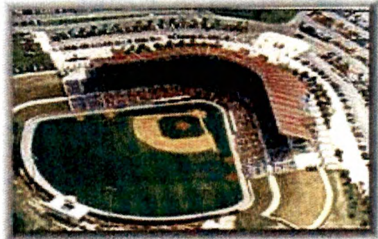
Figure 4-9: Aerial view of the Hoover Met.
