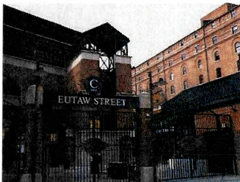
Figure 2-1: Oriole Park at Camden Yards, Baltimore.
