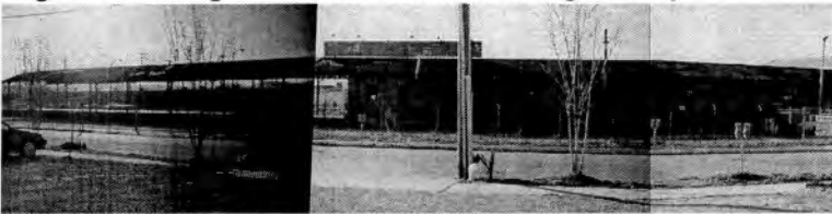
Fig. 28: Existing Abandoned Train Shed
