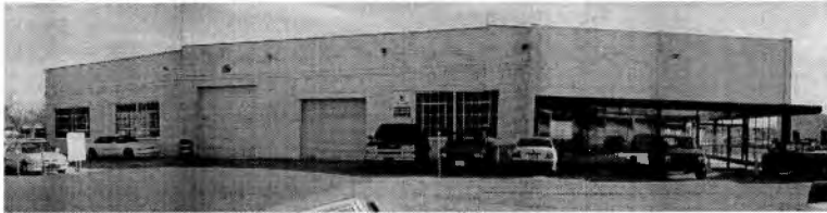
Fig. 26: Existing Abandoned Auto Showroom
