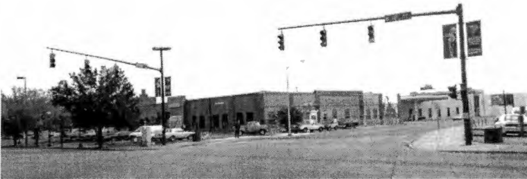
View of Site Looking South Down Broad Street from TVA
