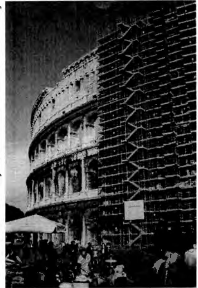
The Coliseum with scaffolding Source: Andy Berry
