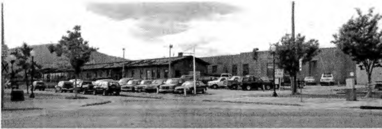
View of Site Looking Southwest Toward the Existing Buildings
