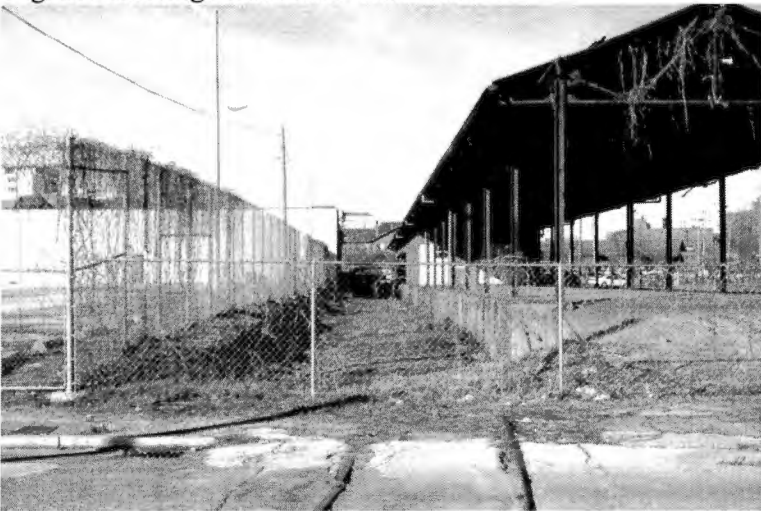
Fig. 29: Existing Abandoned Railroad Bed
