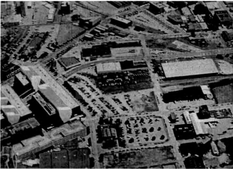
Aerial View of Site Looking Southeast
