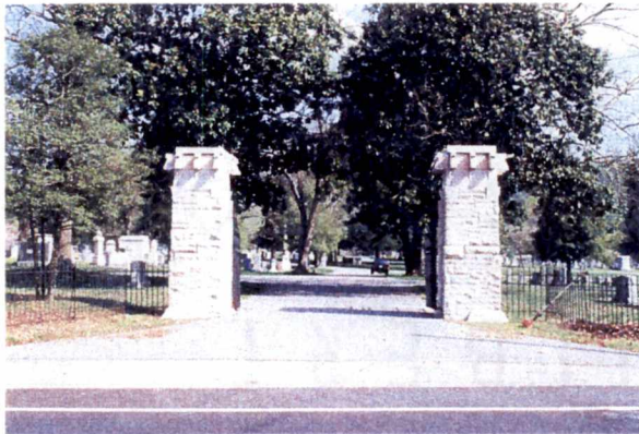
Figure 3.18 Original Limestone Pillars Located at Greenwood Cemetery
