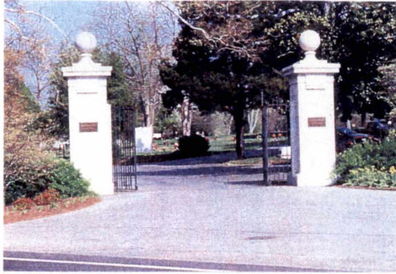
Figure 3.19 Neo-Classical Pillars Located at Greenwood Cemetery (Constructed 1930)
