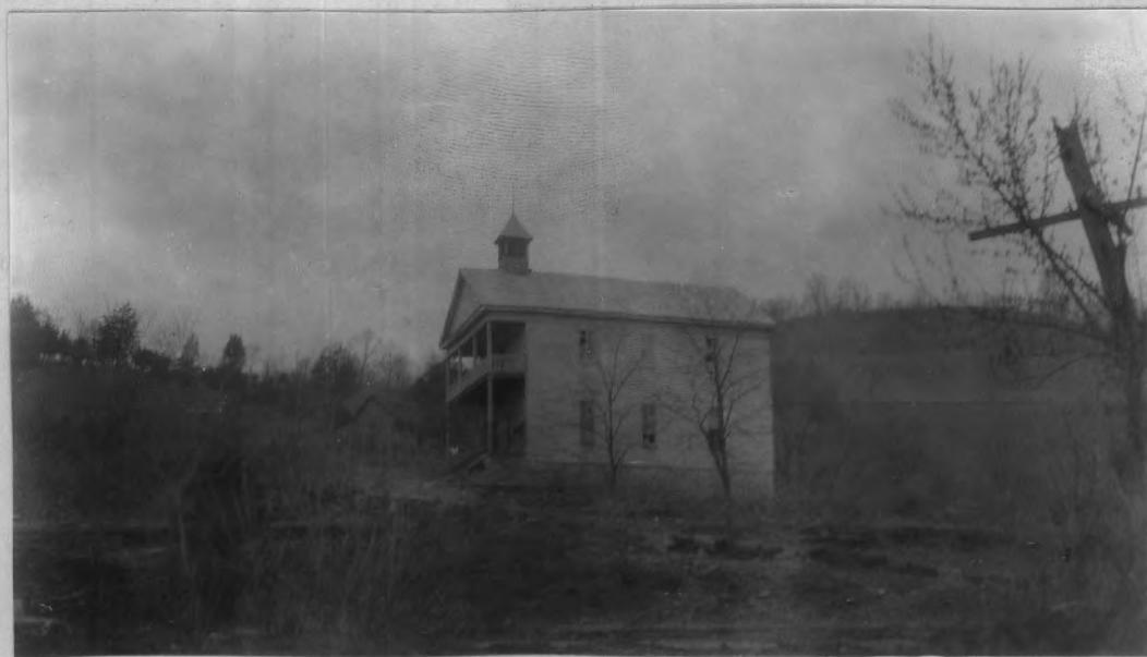
The above building is used by the school, church and Masonic lodge.
