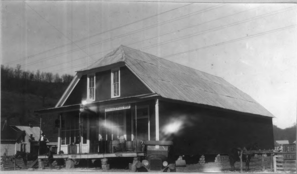
One of the largest country stores in the county
