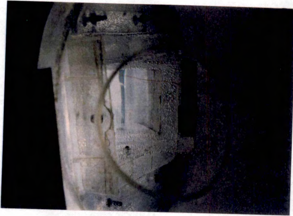
Zone 3, View Upstream into Nozzle Exit
