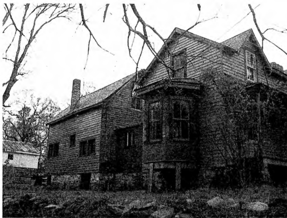
Figure 6. Rear of Uffington House, 2001.
