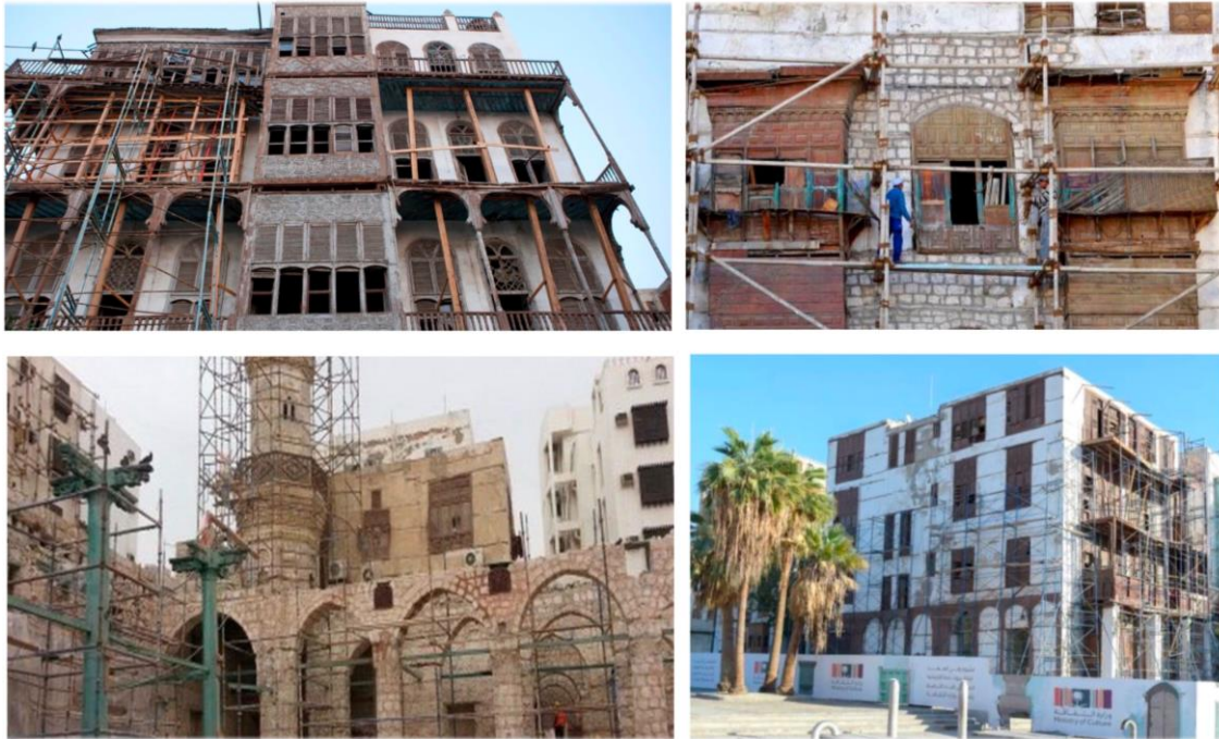
Fig. 06. Renovation work for various buildings in the Al-Balad district.
