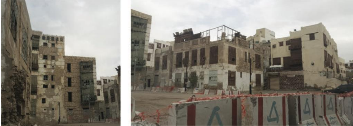
Fig. 01. The deteriorating state of Al-Balad's urban fabric.
