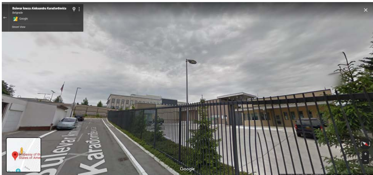
Figure 78. Non-blurred images of the U.S. embassy is at the very end of a cul-de-sac of Bulevar kneza Aleksandra Karađorđevića Street. Google Street View.
