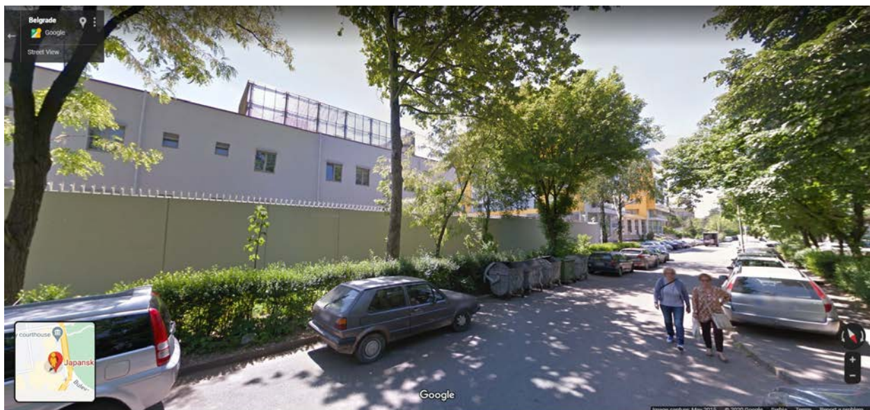
Figure 71. Undisturbed parking alongside the northern parameter wall of the Japanese embassy in Belgrade. Image capture May 2015. ©2020 Google.
