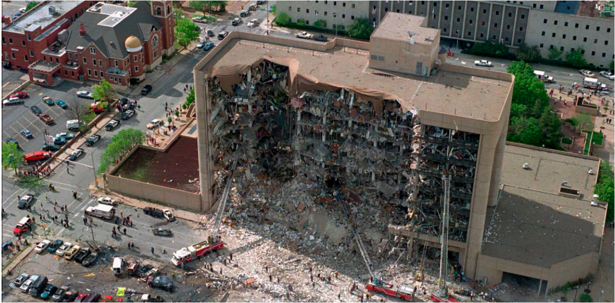
Figure 49. April 19, 1995 aerial file photo, the north side of the Alfred P. Murrah Federal Building in Oklahoma City ( https://www.ksla.com/2020/04/19/sunday-marks-th-anniversary-oklahoma-city-bombing/ )
