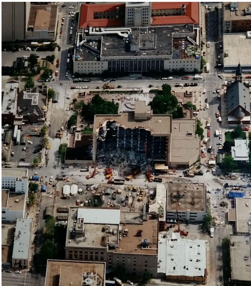
Figure 47. Aerial photo of the wider urban destruction around the Alfred P. Murrah Federal Building ( https://i.pinimg.com/originals/1f/be/d3/1fbed3197b43b2a7f046f16249bc22e0.jpg )
