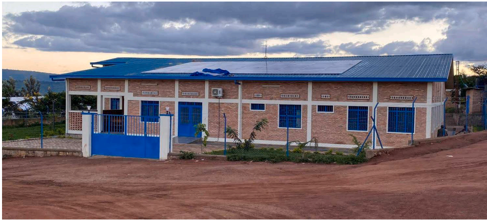
Fig. 1. The health centre at Mahama Refugee Camp with the solar generation on the roof. Photograph courtesy of Arthur Santos and MeshPower Ltd.
