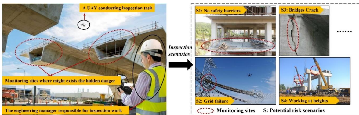
Figure 10: The application of the UAV-based inspection approach in the engineering management
