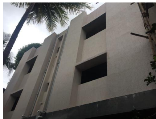
Fig8 b – Ferrocement panels fixed on LGS frame
