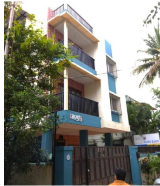
Fig 8c – Full scale construction of G+2 and a completed vila using LGS Ferrocement composite technology
