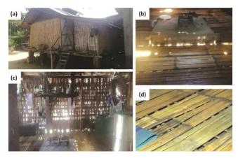
Fig. 9 — (a) Structure made of bamboo (b) fireplace used for cooking and heating (c) perforated bamboo walls (d) bamboo flooring
