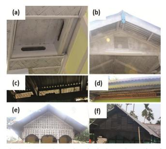
Fig. 8 — (a) Interior opening of attic (b) exterior opening of attic (c) & (d) gap between roof and wall (e) & (f) bamboo shading device
