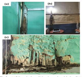
Fig. 3 - (a) Sal wood column (b) interior wattle and daub wall (c) exposed part of wall
