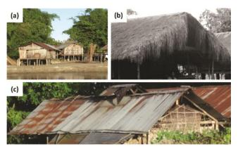
Fig. 10 — (a) Stilted structure built near river bank (b) thatch roof used in older houses19 (c) GI sheet sloping roof used currently
