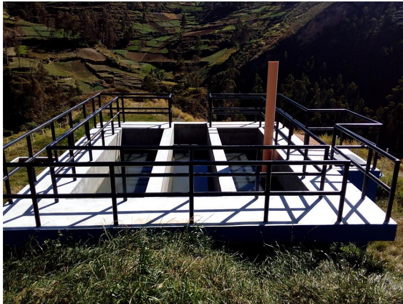
Figura 12 – Tanque imhoff.
