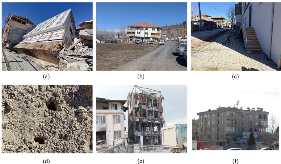
Fig. 18 a An overturned building, b unequal settlement of a building, c settlement of ground, d sand boils, e secondary disaster, f damaged facilities atop a roof
