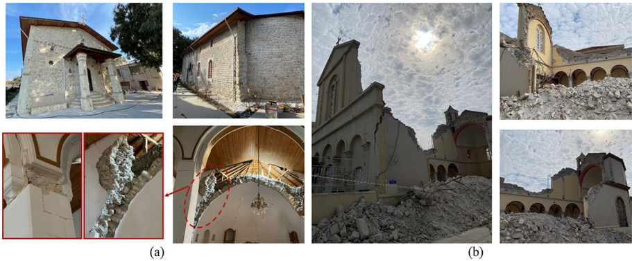
Fig. 37 Damage of churches a St. Ilyas church in Samandagi, Antakya, b Roman Catholic Church in Iskenderun
