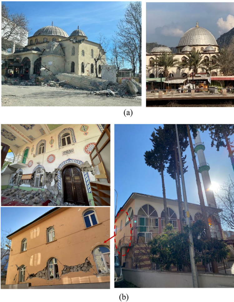
Fig. 36 Damage of mosques a Haci Murat Mosque in Kahramanmaraş, b Merkez Cumhuriyet Mosque in Pazarcik
