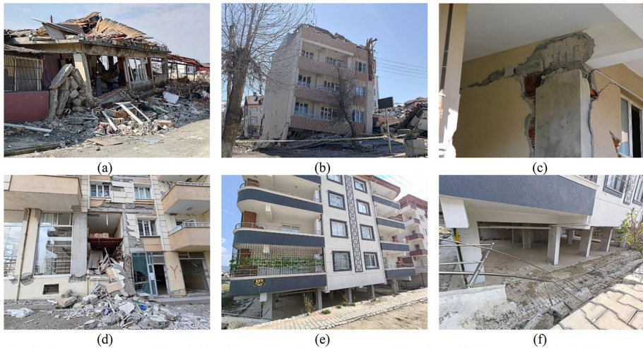
Fig. 19 Structural damages a and b collapsed buildings along a significantly weak direction; c plastic hinges at top and d plastic hinges at bottom of columns, e an almost intact building, and f a close-up photograph of e
