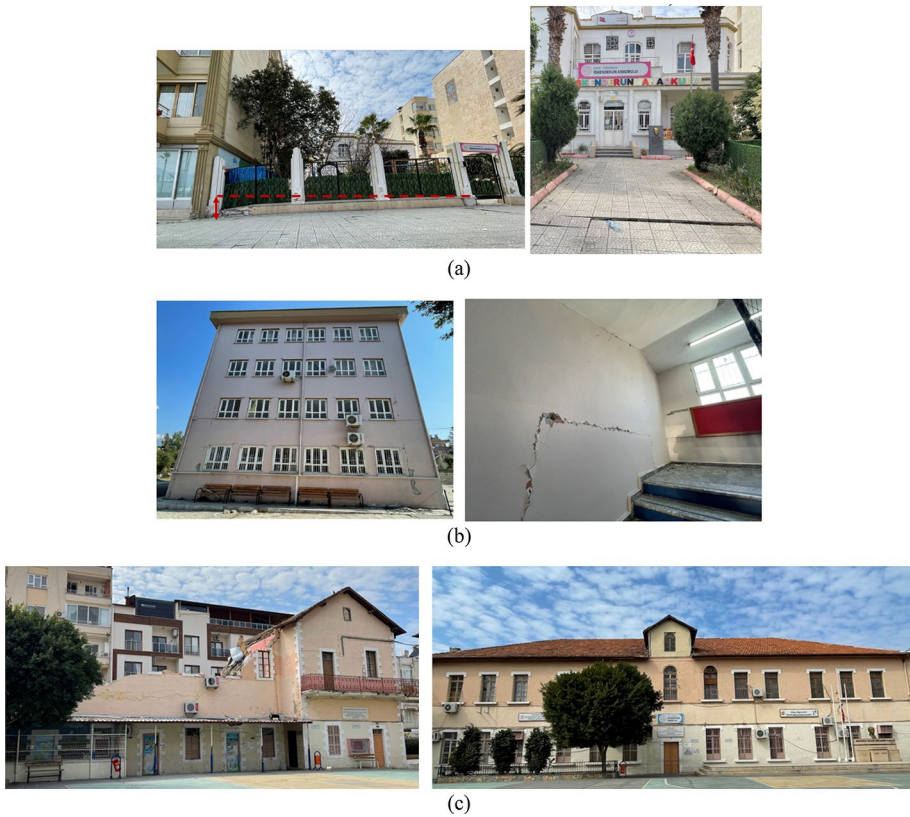
Fig. 35 Performance of schools in Iskenderun a Pre-school, b Retrofitted elementary school, c Unretrofitted elementary school
