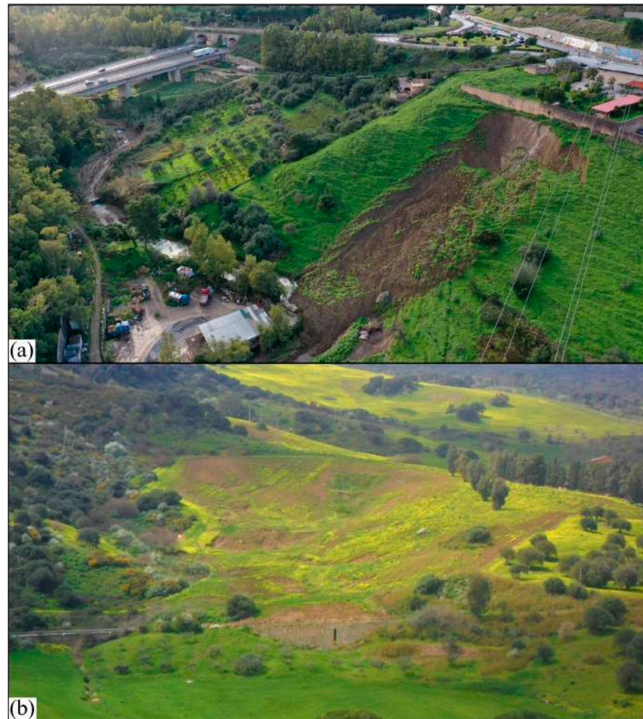
Figure 3. (a) Rotational slide/flow landslide affecting the slope of the A19 motorway; (b) multiple rotational slide/flow landslides affecting the slope of the SS120 national road.
