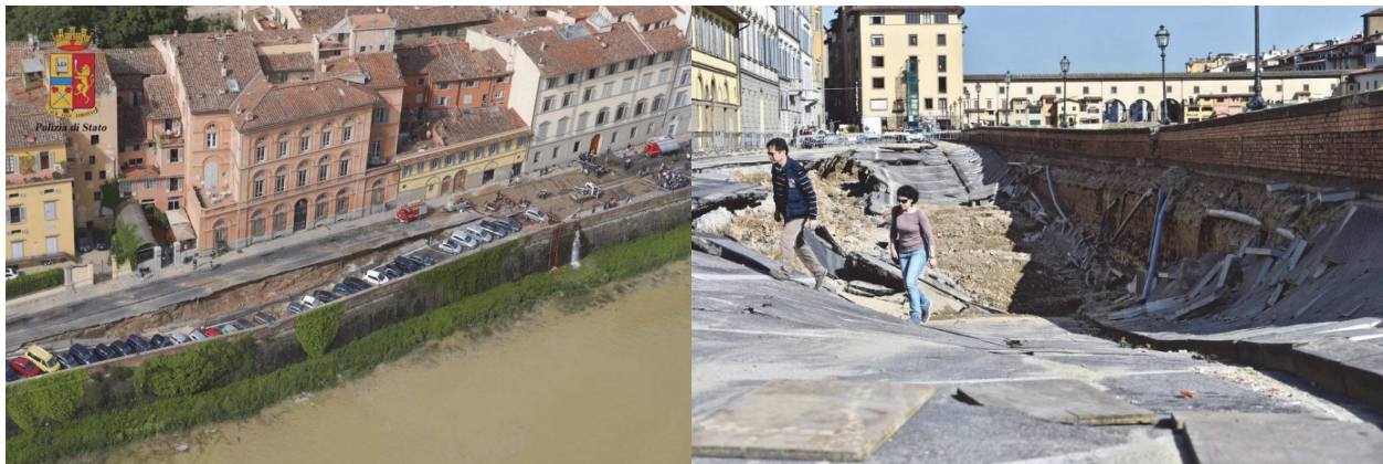
Figure 3: Collapse of Lungarno Torrigiani in Florence (25 th May 2016) as an example of moisture related failure.
