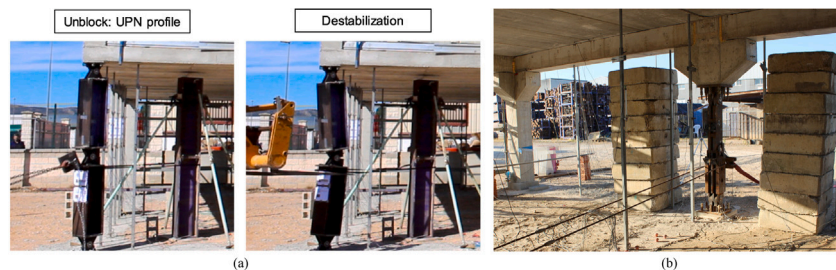
Fig. 13. Dynamic column removal in dummy column assemblies (a) pushing by slight destabilization of the column using a forklift, as reported in [30] and (b) pulling, the cables were connected to a hydraulic jack (test performed at Universitat Politècnica de València [57]).
