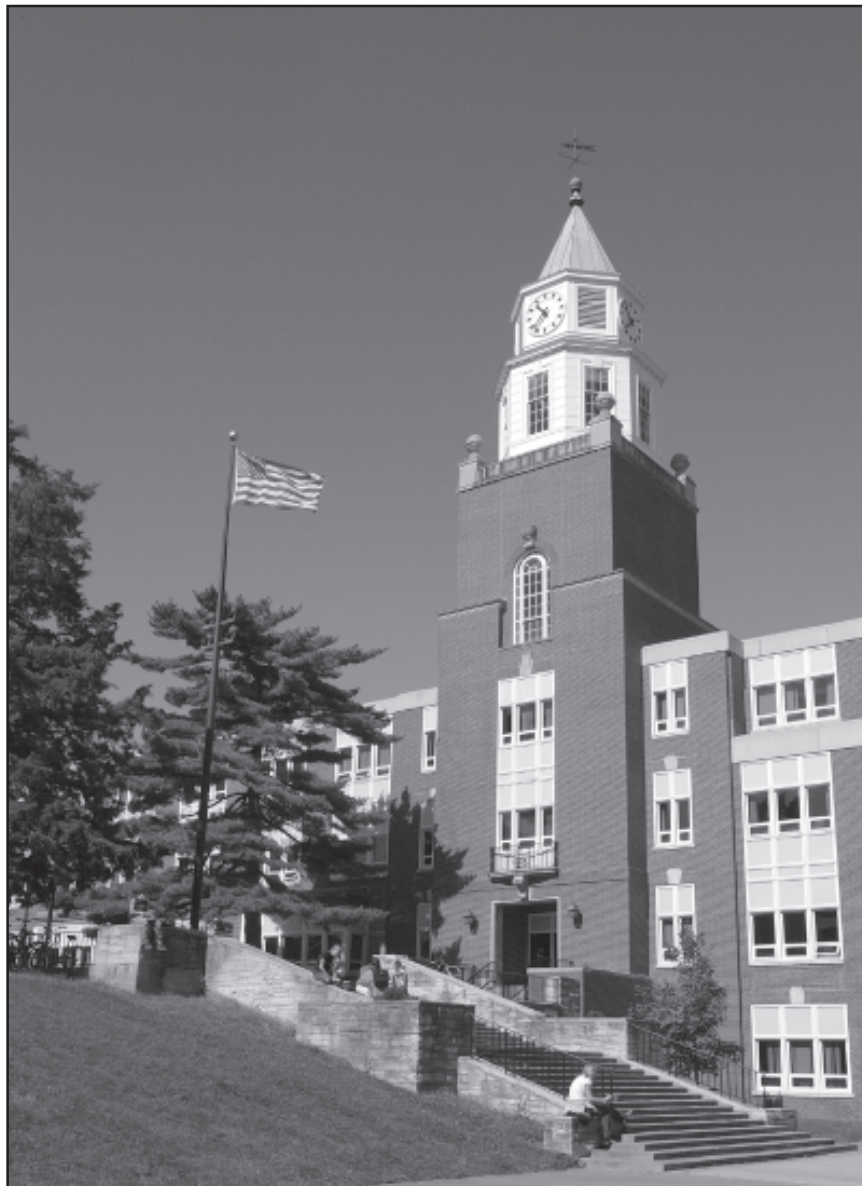
Pulliam Hall, Southern Illinois University Carbondale
