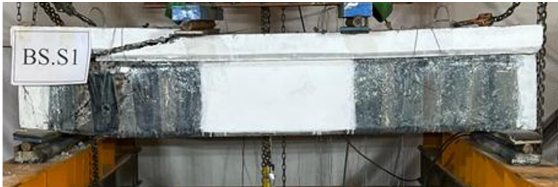
Figure 15. Pattern of cracks in sample BS.S1
