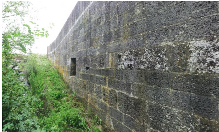
Figure 12. Spandrel wall of Halilviran Bridge
