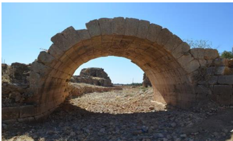
Figure 10. Damage arch of the Dara Bridge
