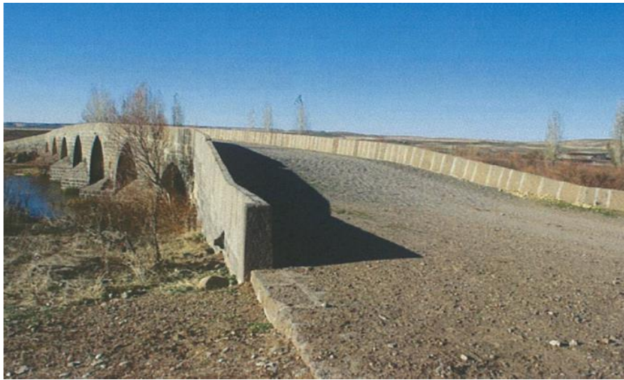
Figure 14. Halilviran bridge roadway
