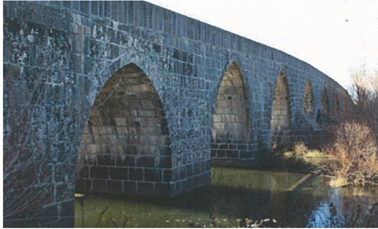
Figure 11. Arch of the Halilviran Bridge
