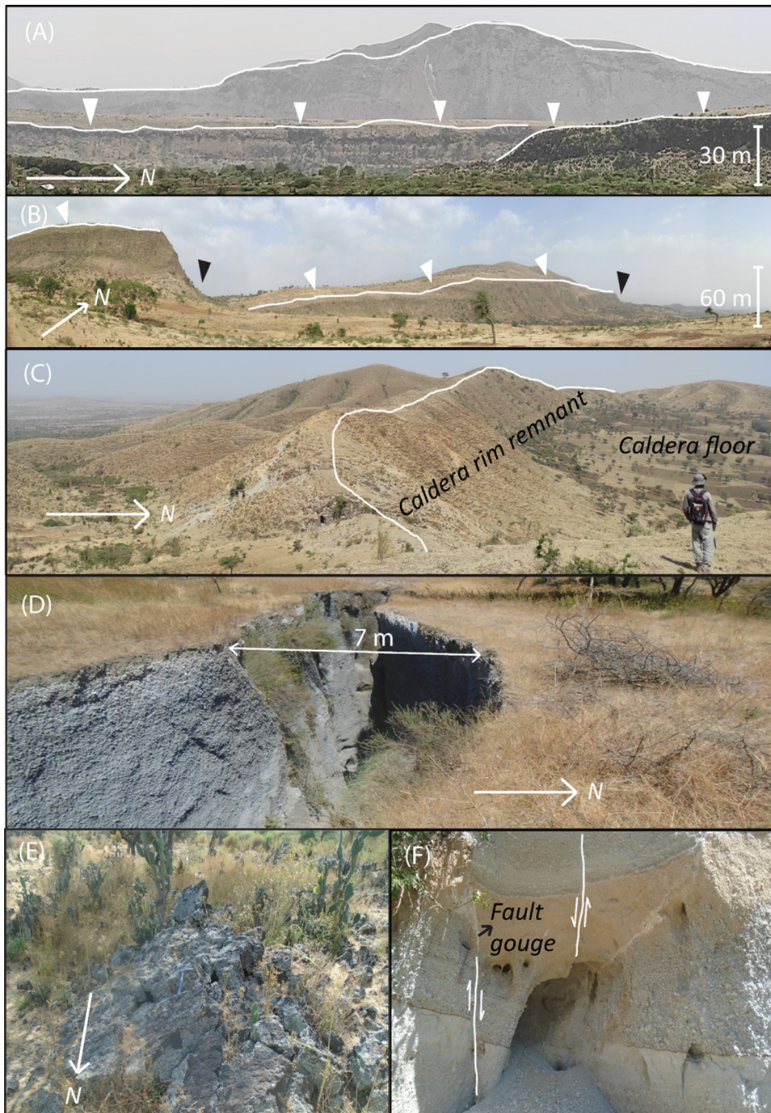
Figure 4: Field photographs of volcano-tectonic structures in the BBTM volcanic system. The geographic North is indicated by a white arrow on each photo. [A] Regional NE–SW trending border fault, showing fault termination. [B] Regional NW–SE trending cross-rift faults cut by NE–SW trending faults (black arrows). [C] Ring faults located in the southern part of the BBTM volcanic system. [D] Open fissure in a pyroclastic deposit located North of Werdi edifice. [E] Eruptive fissure located North of Miesa. [F] Two opposite dipping faults trending NW–SE in pyroclastic deposits.
