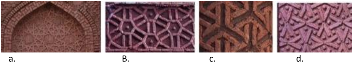
Figure 2.18: 12-point, 6-point, abstract 6-point, and 8-point geometrical patterns from Tower of Kharaqan in Qazvin
