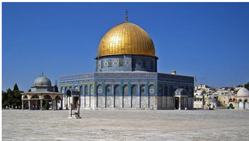
Figure 2.23: The Dome of the Rock( Qubbat al-Sakhrs), Umayyad Stone masonry, wooden roof, decorated with glazed ceramics and gilt aluminium and bronze dome
