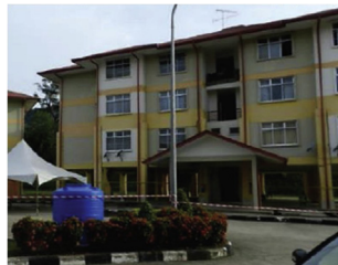
Fig. 6. Selected reinforced concrete building.
