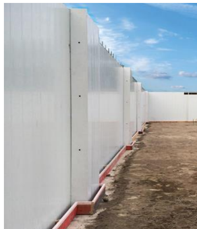
Figure 1-2 Smooth finish of AFS formwork system
