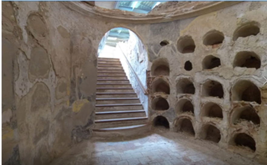
Figure 5. Detail of the stairs to the crypt
