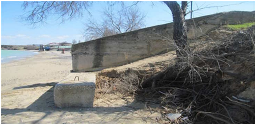
Fig. 10. Coast protection of the village of Uglovoye.
