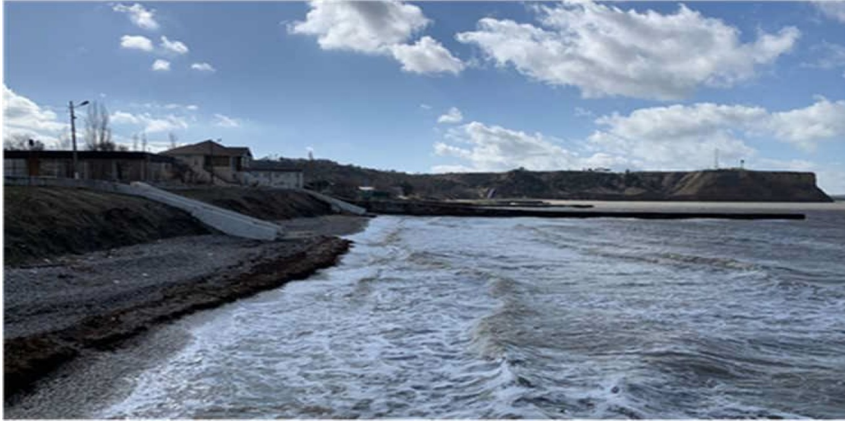
Fig. 9. Coast protection of the boarding house "Peschanoe" and the children's health camp "Yuzhny".
