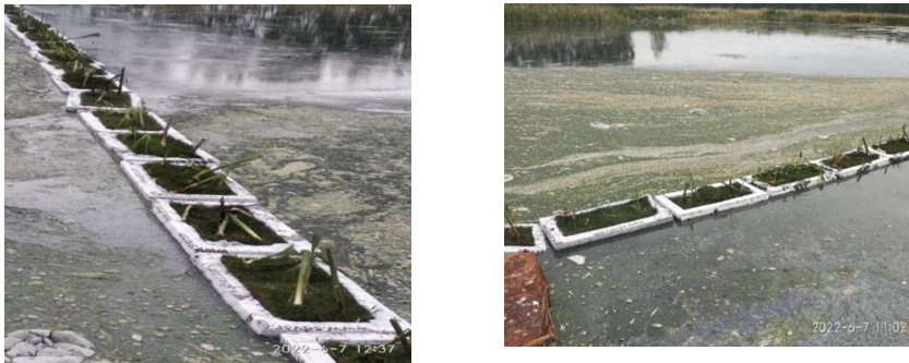
Fig. 7. Installation of the bioplate
