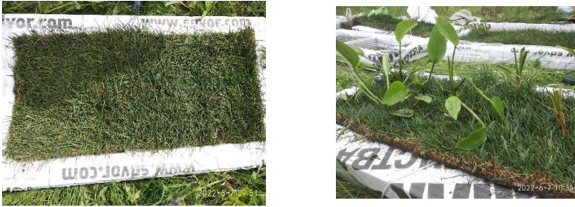
Fig. 6. Stages of installing the bioplate
