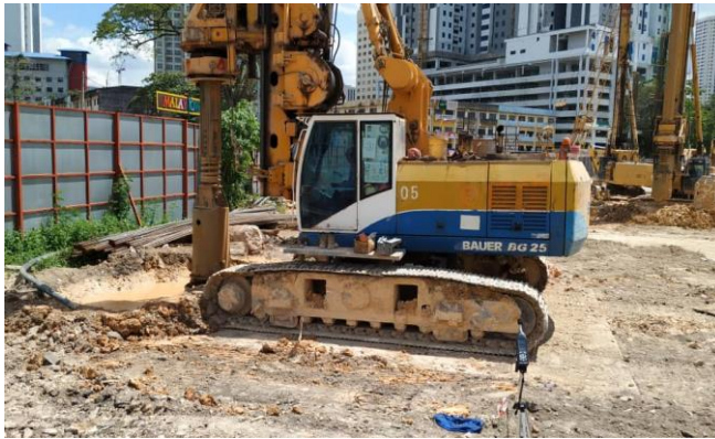
(a) Piling Activity
