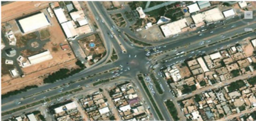
Figure 4: Aerial image from the Maps app of the Al-Salam intersection.
