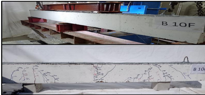
(d) Crack patterns in the tested extended continuous beams at the failure stage (BF10).
