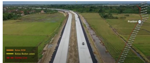
Fig. 1. Aerial photography with a drone on Semarang-Demak Toll Road section (PT PP).
