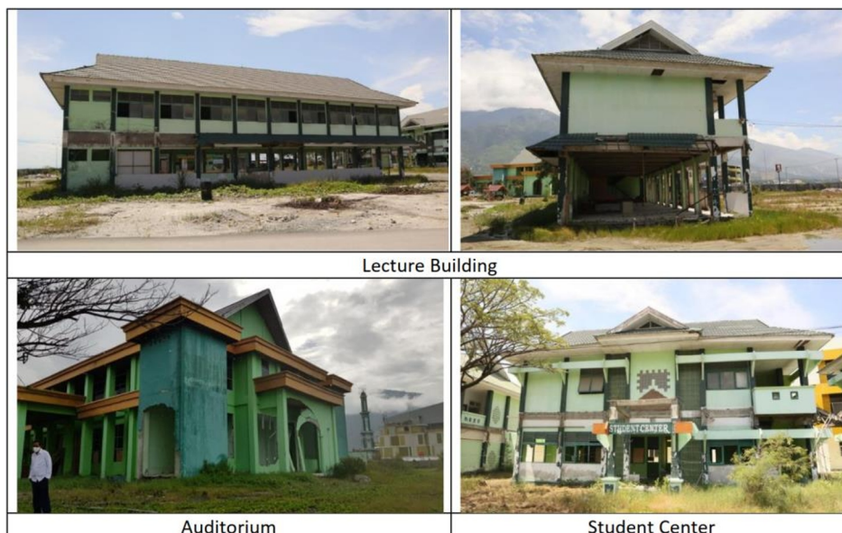
Fig. 2. Examples of severely damaged buildings at IAIN's campus 1 [1].
