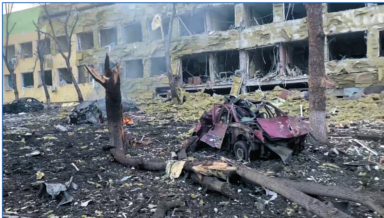
Figure 1. A children's hospital in Mariupol was destroyed as a result of a Russian airstrike ( www.pravda.com.ua/news/2022.03.9.7329805 )
