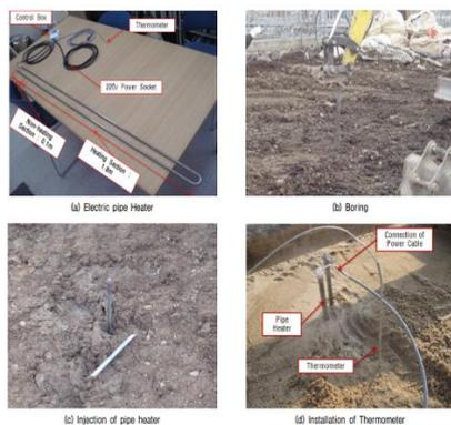
**Figure 1.** Soil improvement using Heaters (Park et al., 2012)
