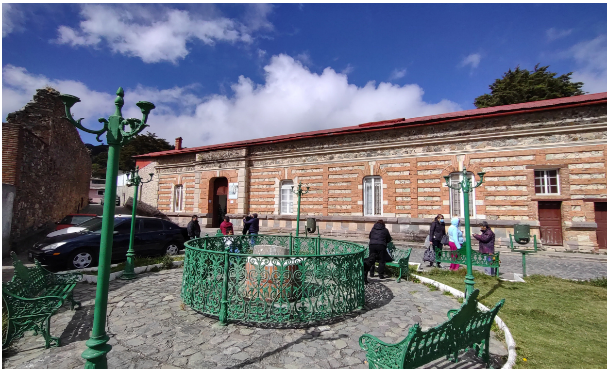
Figure 6. The Main Facade, facing south along Hospital Street, photograph by Author.
