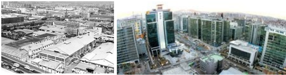
Figure 10. Past & Current View of Guro Industrial Complex
