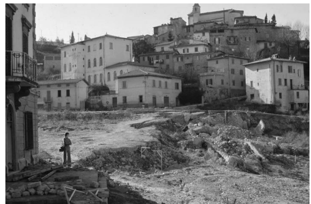
Figure 3. Demolition of the lower part of the village.
