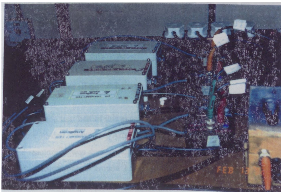
Figure 3.6: SBR System and Transmitter/Amplifiers Assembling Pictures
