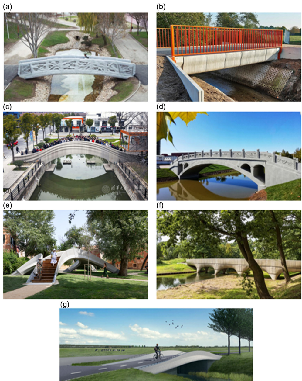
FIGURE 2 3DPC footbridge projects: (a) Parque de Castilla (credit: Institute for Advanced Architecture of Catalonia, IAAC); (b) Gemert (credit: Marc Zoutendijk); (c) Wisdom Bay Park (credit: Tsinghua University); (d) Zhaozhou (credit: Xinhua); (e) Striatus (credit: naaro); (f) The Bridge Project (credit: Municipality of Nijmegen); and (g) N243 route (credit: Witteveen+Bos).
