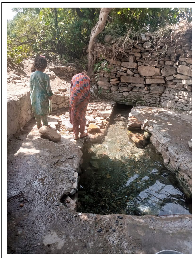
Figure 3. Randa Cheena, near Nagoha, Swat Valley, Pakistan, illustrating the engineering traditionally undertaken to improve springs (photo courtesy: Izhar Khan).
