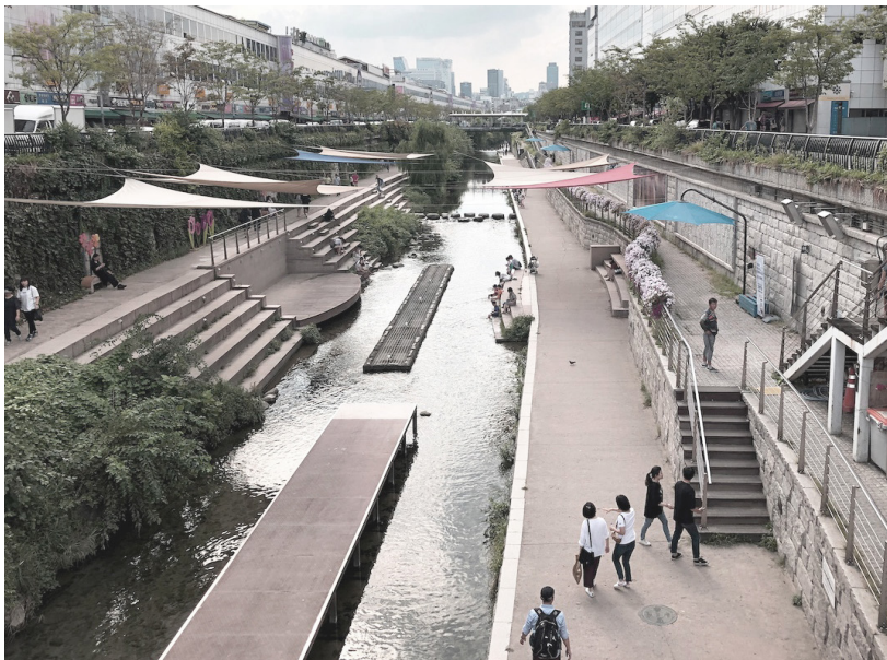
fig. 23: Variety of features in the riverbed, access, isolation from road on street level
