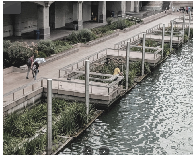
fig. 33: Chicago river, top: first settlement around it in 1832, middle and bottom: the riverwalk of Chicago, after its completion in 2016
