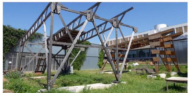
FIGURE 43 Structural prototypes in the courtyard. Source: Compiled by authors.
