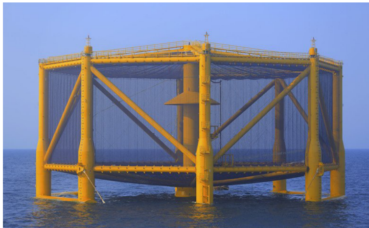
Figure 5.2: Offshore Rigid Structure - Shenlan.
