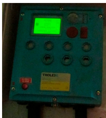
Figure 1. Trolex fixed gas monitoring station.
